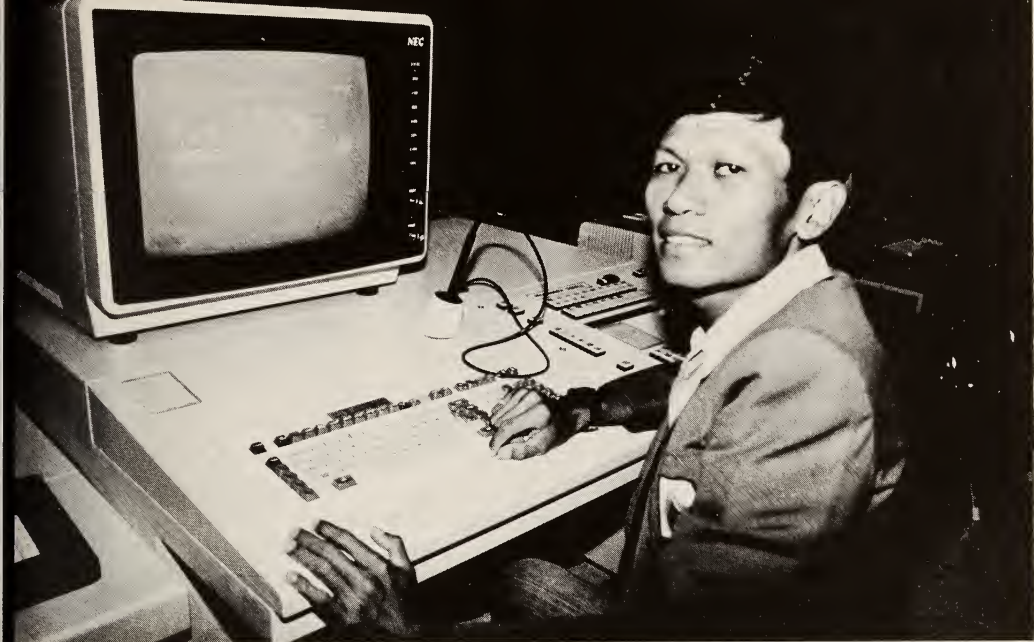
Technician at the natural gas-fueled Ban Pakong power-generating station southeast of Bangkok Courtesy World Bank
